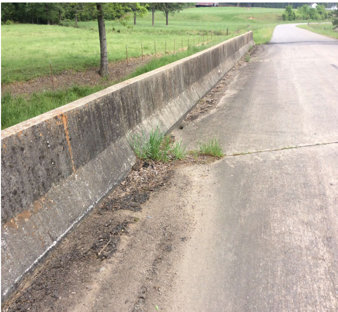
PHOTO 1 Description Dirt, debris and vegetation along the Lt and Rt gutters.
