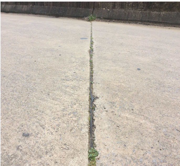
PHOTO 1 Description Deck joint sealant is deteriorated and leaks water on the caps.
