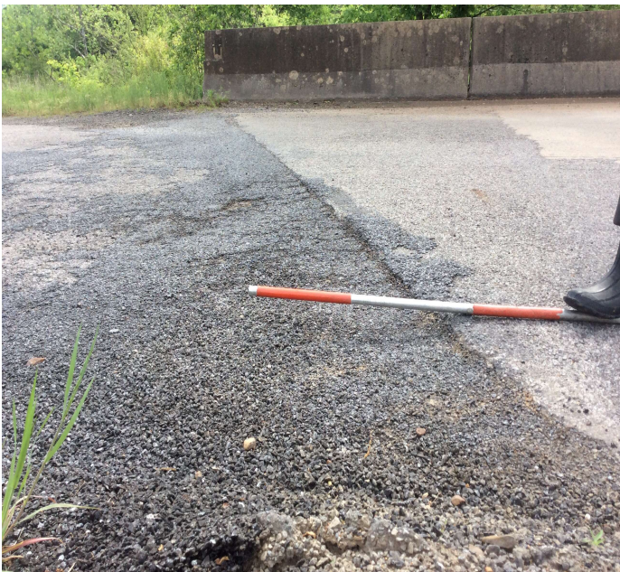
PHOTO 1 Description The North approach road has settlement with asphalt cracking and potholes at the bridge end.
