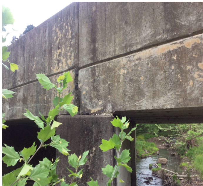
PHOTO 1 Description Minor spalling in the edges of the deck and in the caps of Bents # 2 & 3.
